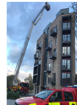
Nov 2021 - crews visit new high rise blocks
